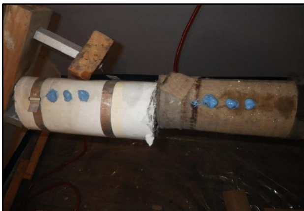
14. Wonder Fill, a blue encasement and encapsulant mastic, was used to fill the voids created by the collection of the samples from the asbestos-containing pipe insulation.
